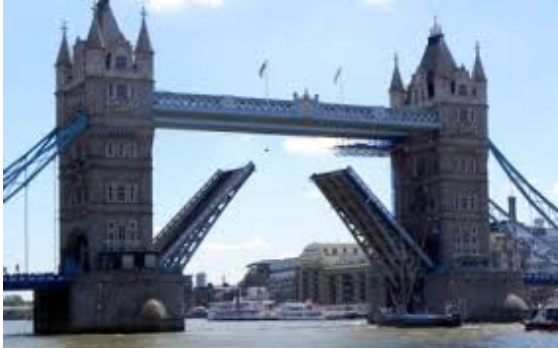
Figure 1 – Drawbridge, span raised as two halves.
